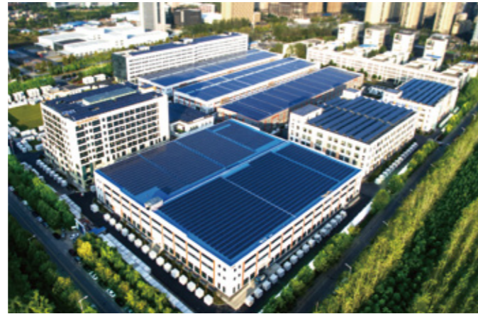
PV+ESS+Charger station in Sungrow HQ in Hefei, China
