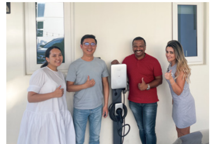
Residential EV charging station in Dubai, UAE
